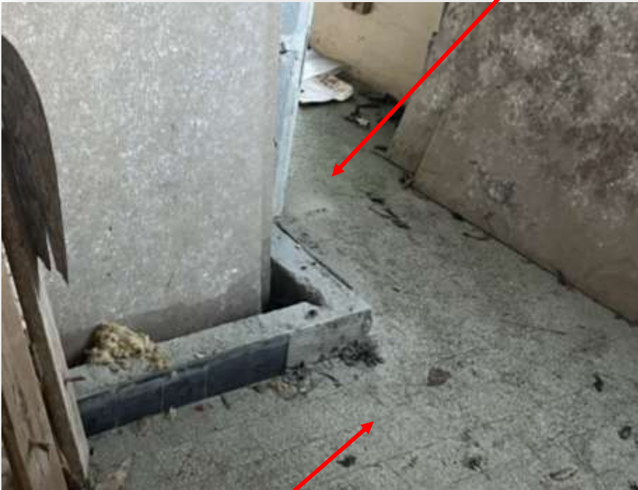
Railway Power Station
