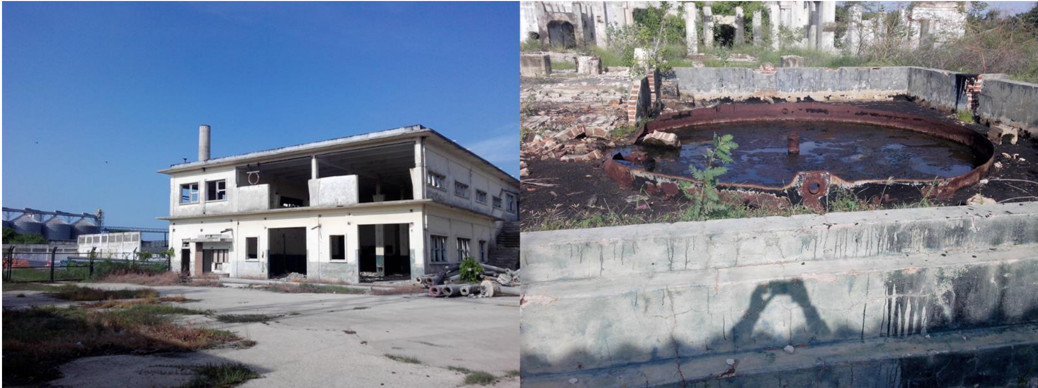
Abandoned power generation facilities
