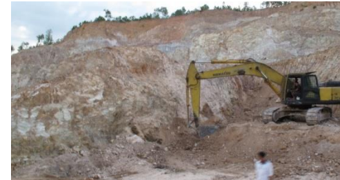
Obtaining clean back fill material
