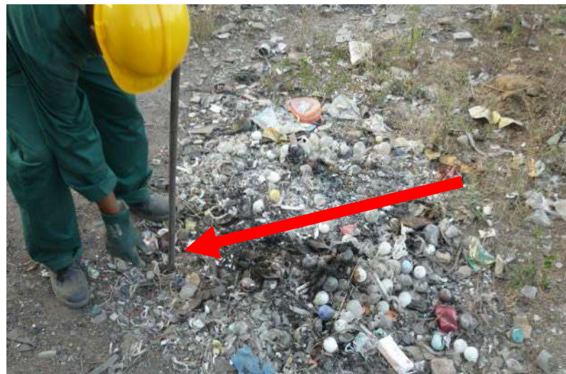
Installing gas extraction probe
