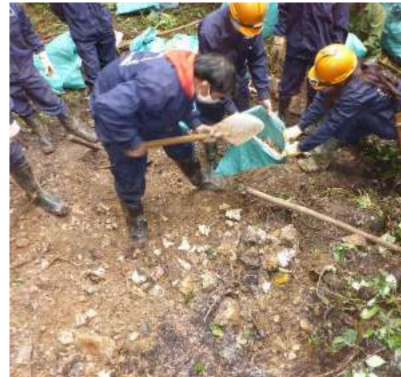
Excavating soil mixed with DDT
