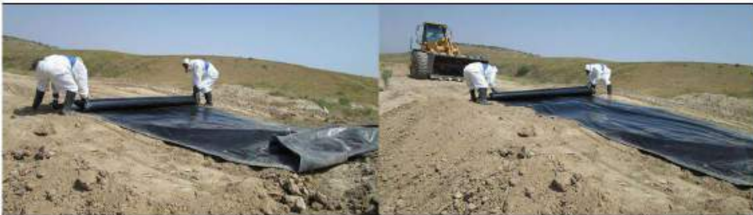
Figure 3 Application of HDPE plastic as topcover for the hot-spots
